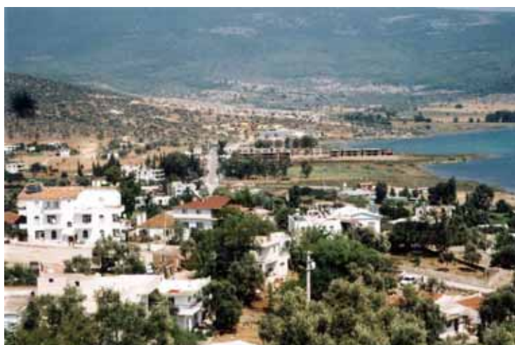
Fig. 5. Iasos, construction area of a new holiday resort on the back
