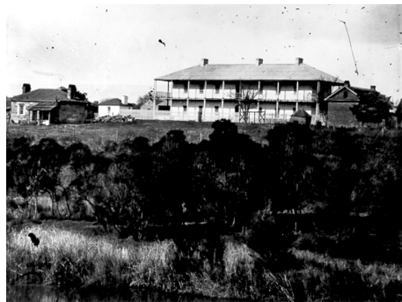
Fig 11: The Hospital as it looked in the 1870s with the Parramatta River in the foreground (DPWS archive)
