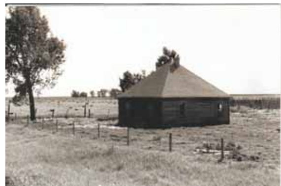
Fig 5: Cultural: This is one of the early settlement houses near Stirling. Typical building patterns for the Mormons included steep pyramid roofs.
