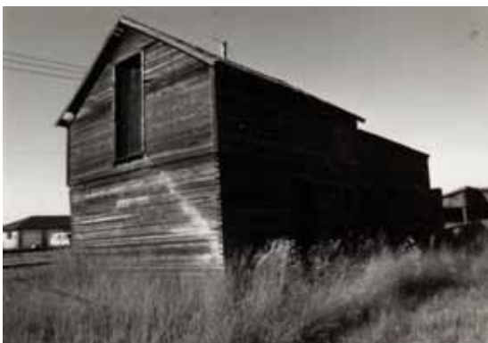
Fig 4: Cultural: Granaries and barns built on the homestead were typically constructed of stacked square-edged timber to ensure support and were usually left unpainted.
