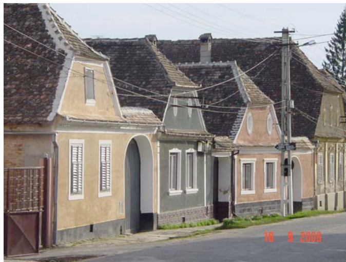
Figure 2. Intact saxon houses in Biertan (Birtäl), protected as world heritage
