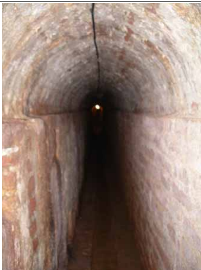
Fig 11 Drainage tunnel from the gaol.
