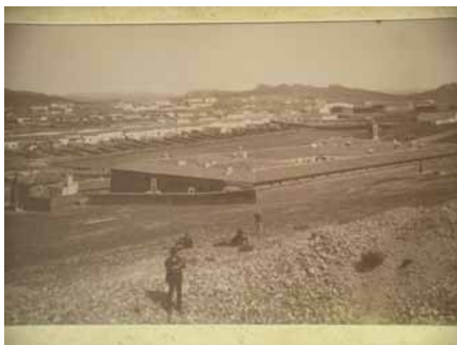
Fig. 13 Gaol before its demolition.
