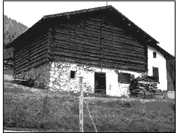
4. Example a building with the first level in masonry and the second level in wood
