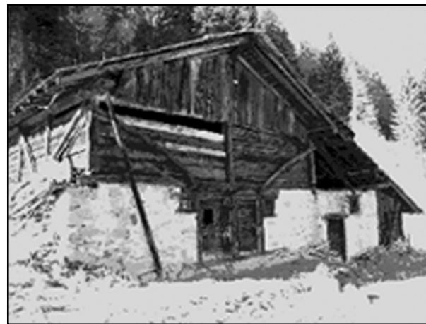
5. Building in framed system on the first floor.
