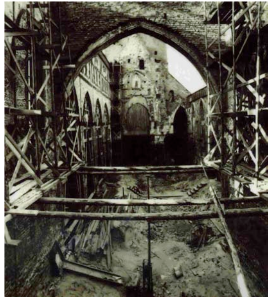
Picture 1. State of Church before restoration.
